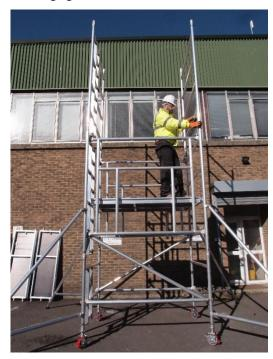
**8)**Fit 2 more AGR's to the end frames, with the top claws on the 10th rungs, lock the AGR's in place as in step 5. Fit a trapdoor deck on the 8th rung, with the trapdoor in line with the one below. Place a fixed deck on the 8th rung next to the trapdoor deck. The tower now has a platform height of 4.2m. If finishing at this height, move on to step 10. If greater platform height is required, repeat steps 7 and 8 until desired height is achieved.
