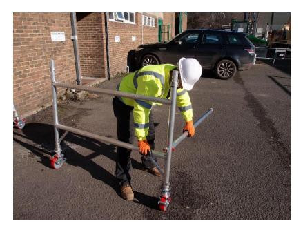
**3)**Position the second end frame as shown and fit the other end of the horizontal brace on to the vertical, just above the bottom rung. Fit a second horizontal brace on the bottom rungs on the other side of the frames to square the tower.
