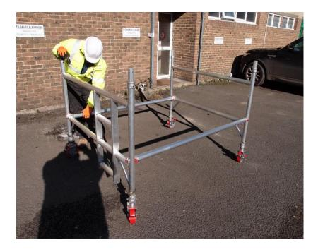
**4)**Fit 2 additional end frames ensuring ladder sections line up and check the frame interlock clips are engaged. Fit 2 diagonal braces (blue) in opposing directions, from the 1st rung to the 3rd rung on the opposing side. Diagonal braces should be positioned approx. 80mm inboard of the frame verticals. Ensure the frames are vertical and level by checking with a spirit level and setting the adjustable legs as required.
