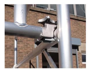
If clear access to the ladder is required, braces may be re-positioned as shown. Reposition braces to original location before moving tower.
