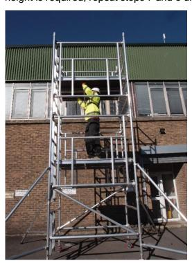
**9)**Continue to add pairs of end frames, AGR's and decks as shown in previous steps, until the required height is reached
