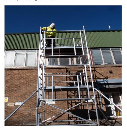
**10)**Fit toe boards Fold over platform making sure location bracket fits securely over platform hooks.
