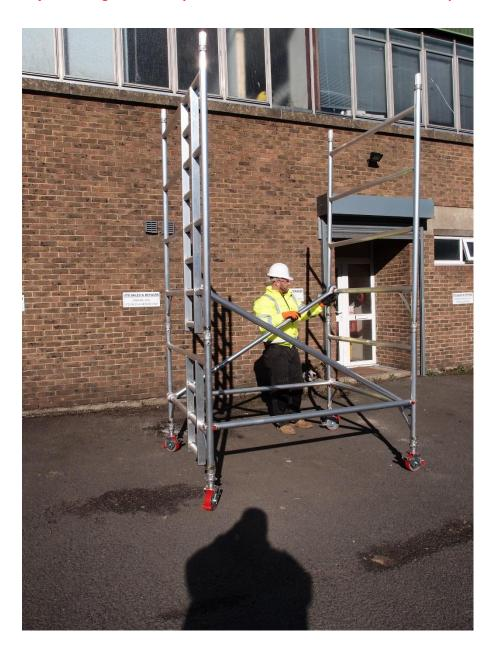
**5)**Fit a Cam-Lock AGR on each side of the tower. The bottom of the AGR must be fitted to the 3rd rung of the tower, as shown. The AGR should be placed up against the end frame verticals.
