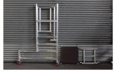
2. OPEN MAINFRAME ENSURING LOCKING JOINT IS SECURED
