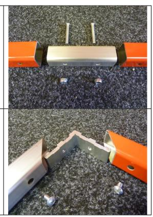
Slot the 2x L" shaped vertical metal rails with straight cut at the top into the T shaped joints on the underside of the red handrails. Tighten 1x bolt and nut horizontally through the T joint and vertical rail.
